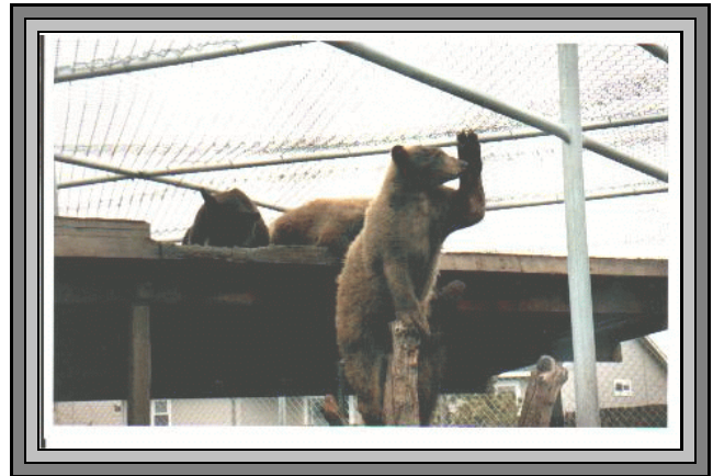
Before reinforcing the chain link roof
