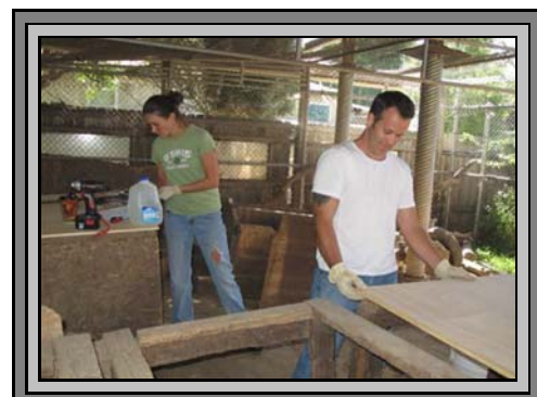
Clint & Tennyson starting to replace all the roofs on the dens
