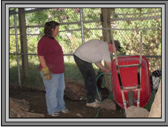
Melanie & Dennis getting ready to mix cement to do all the cement work
