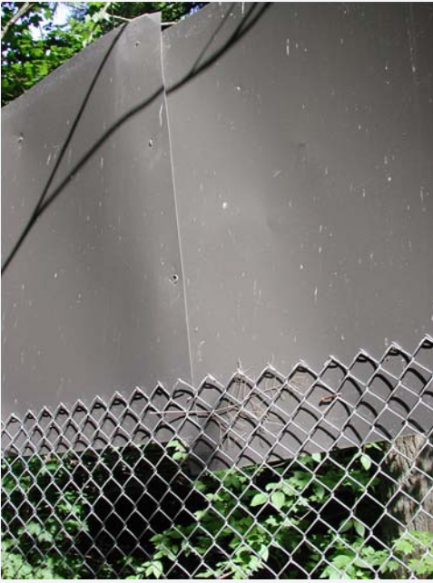
Figure 4. Heavy gauge metal sheeting mounted above chainlink.
